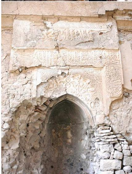
**Photo 6:** Hasankeyf, Koç Mosque. The walls and decoration are endangered from damage and collapse. The building needs immediate conservation treatment.
