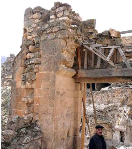
**Photo 5:** Hasankeyf, artukid gate to the upper town. A started conservation treatment has not been finished. The gate in some sections is still endangered from collapse and need further conservation.
